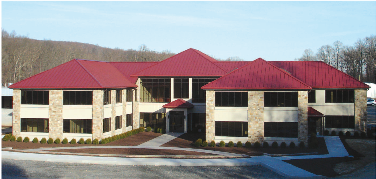
PSI's new worldwide headquarters at the new location in Elverson, Pennsylvania. The office is 23,000 square feet, the factory is 210,000 square feet.
